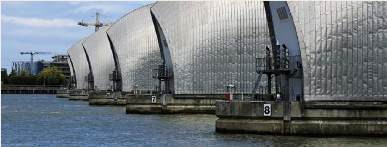
The Thames Barrier works to hold back storm surges and high tides protecting 1.3 million people.
